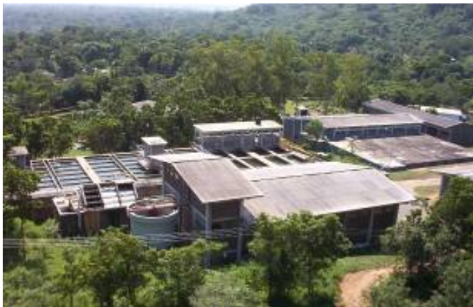
Kantale water supply plant in Trincomalee
